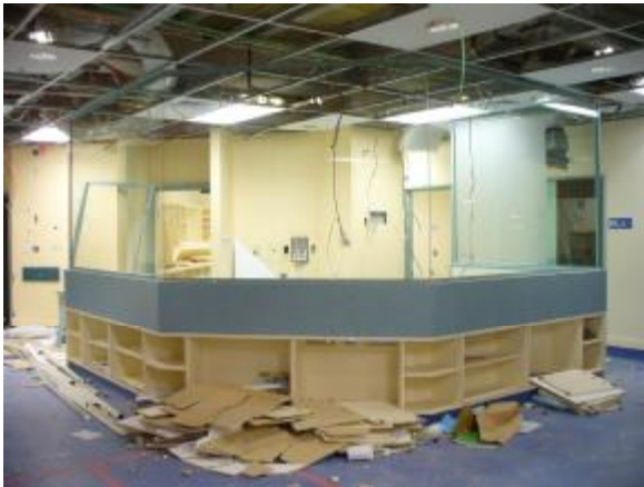
June 2007 - Demolition of old CCU
