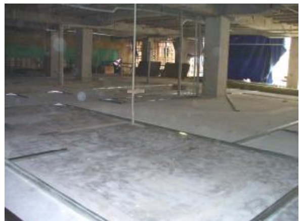
September 2007 - Rooms for the new ICU are being framed
