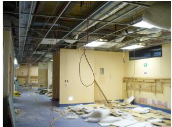
June 2007 - Demolition of old CCU
