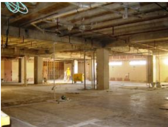
July 2007 - Demolition is complete
