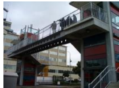
The Kaumatua lead the way for the blessing of the over-bridge.
