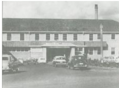
The front entrance of the Hospital – early 1950's
