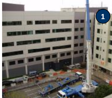
The crane is in place
