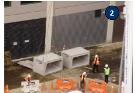
Setting up for the lift
