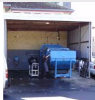
The waste compactor will be moving to the outside of Building 30
