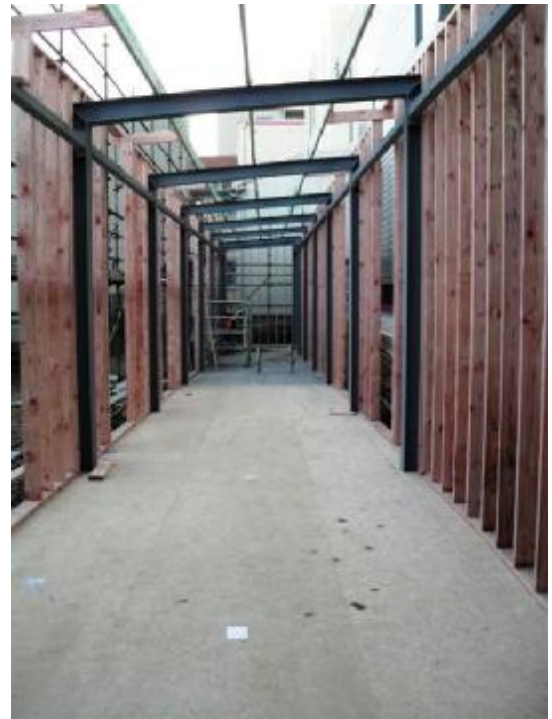
Inside the new link
