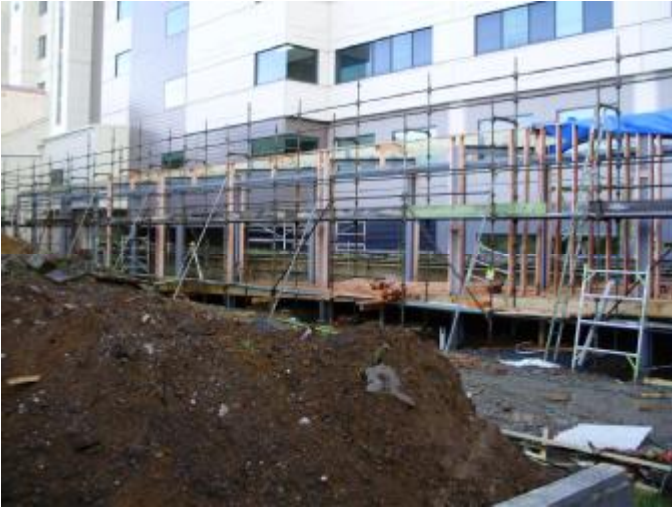
The temporary link is taking shape
