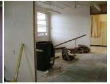
Demolition works are complete for the new Mail Room
