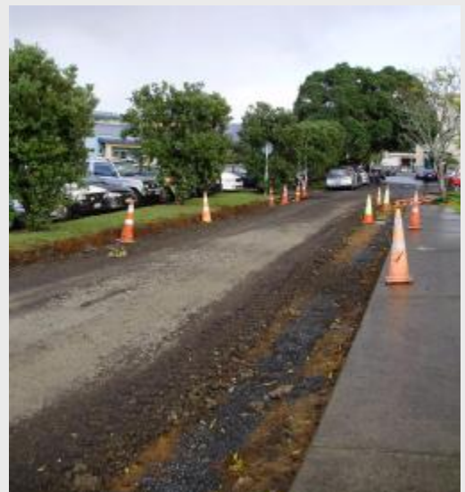
Upgrade of the ring road
